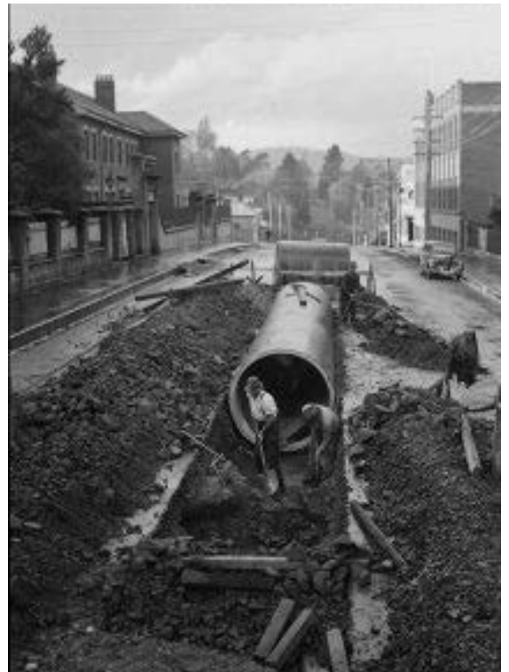
Installing an air raid pipe shelter and trench, Hobart.
